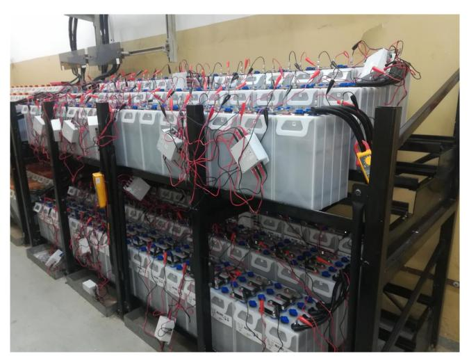
Application case with 21 Remote Measurement Modules (85 cells).
